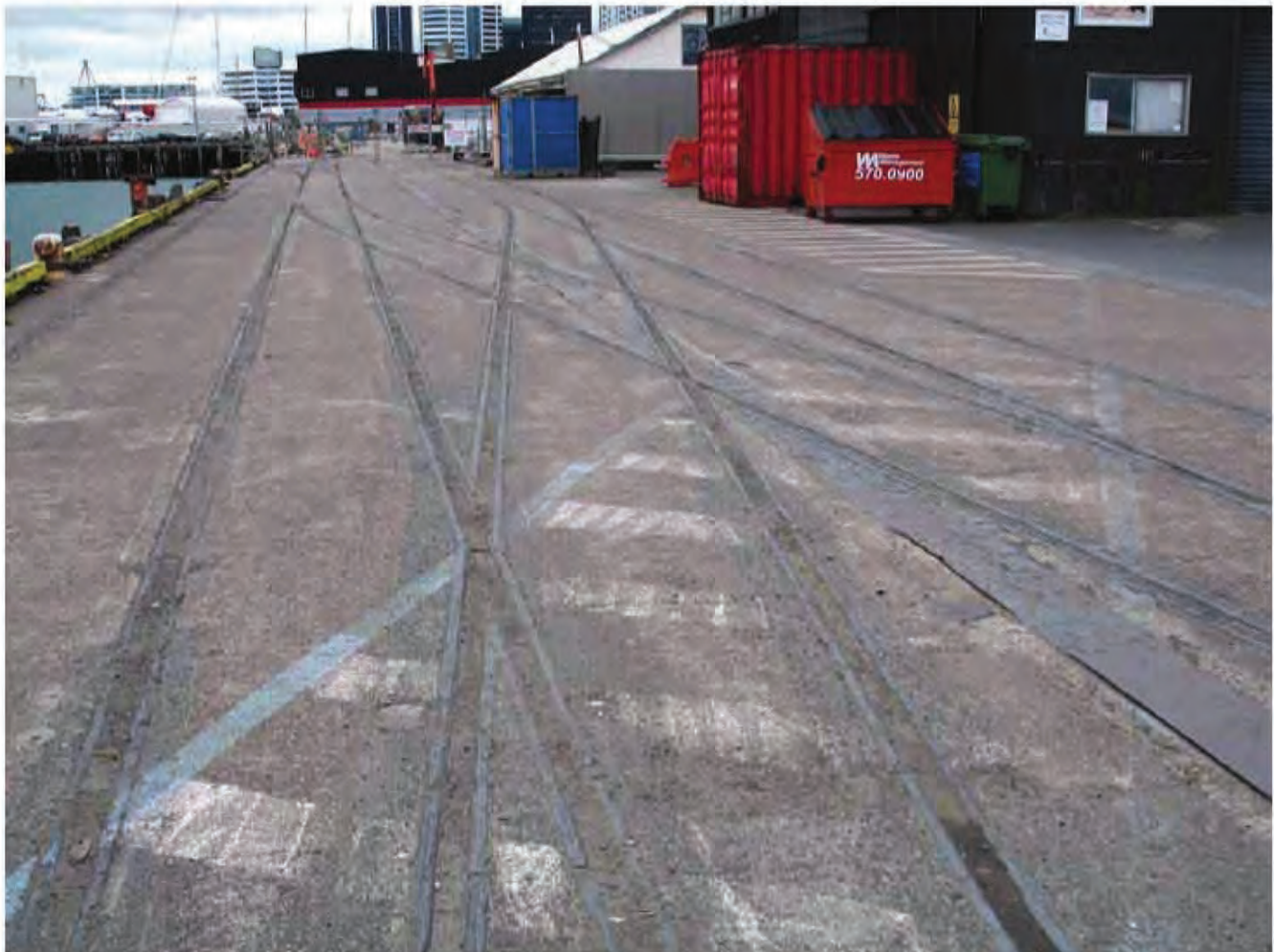
Crane and rail tracks exposed in surface of North Wharf.
