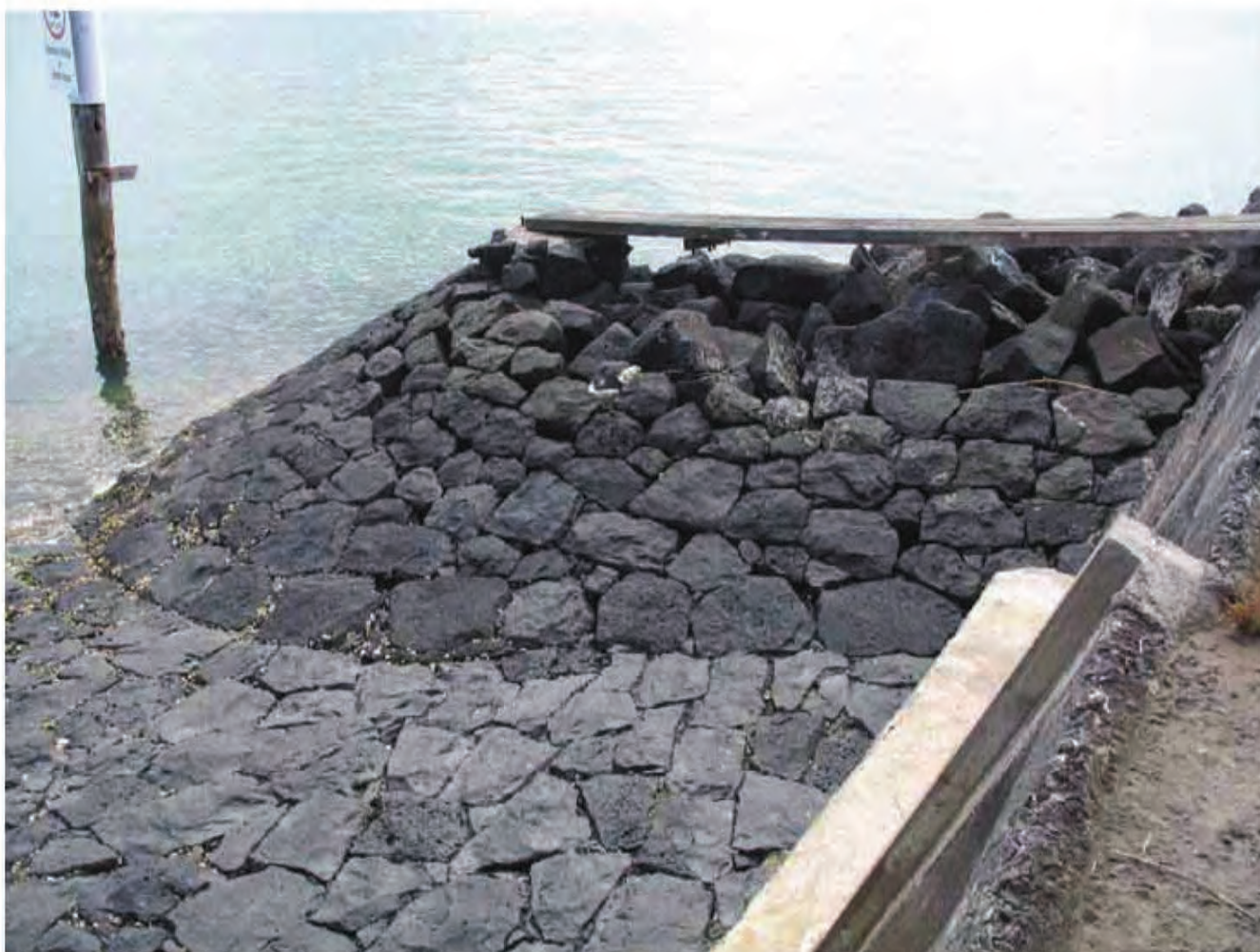
North end of haul ashore - start of rip-rap revetment.
