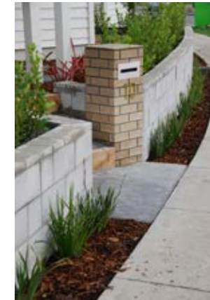
Concrete block retaining wall to front boundary with planting to screen.
