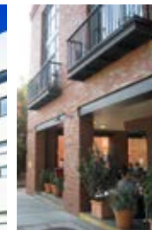
Building line variation
