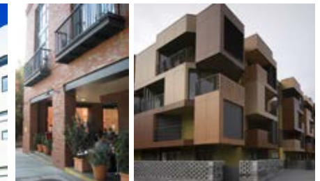
Building line variation
