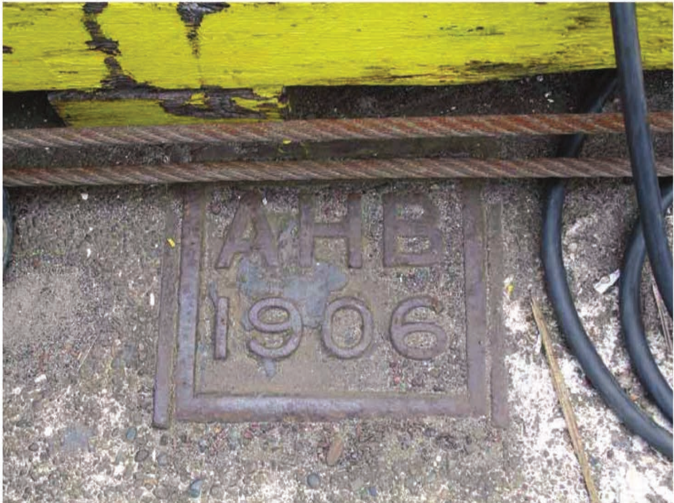
Service cover, North Wharf.
