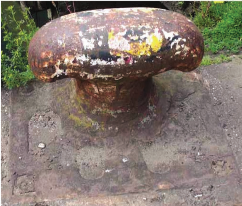
Type L (top, North Wharf) and M (below, Wynyard Wharf alignment) bollards.
