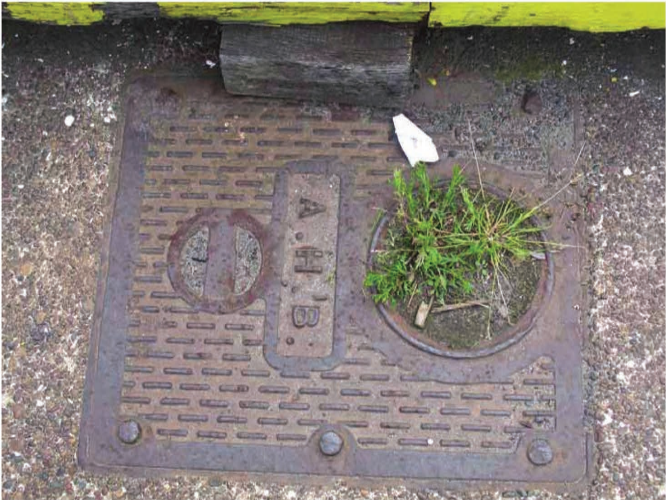
Cast iron fitting (probable davit base), North Wharf.
