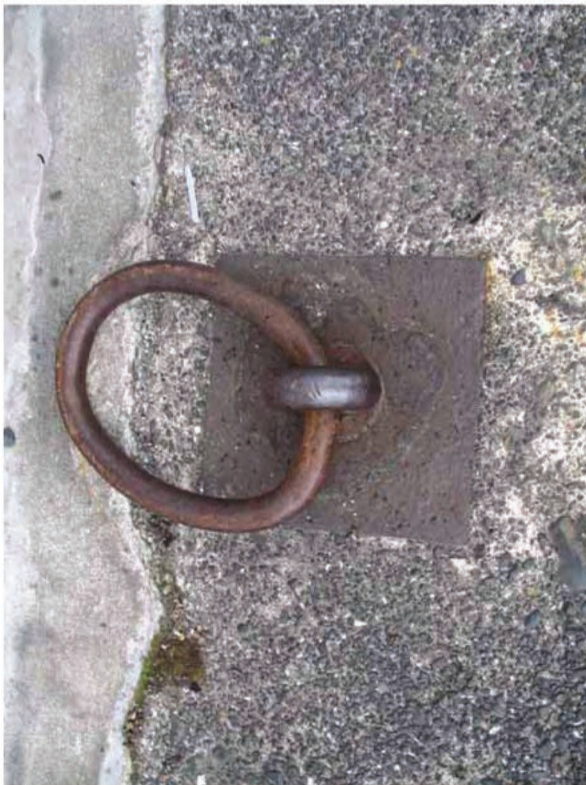
Exposed aggregate surface of Julian's wall (right) with eye-pin and ring fitting.
