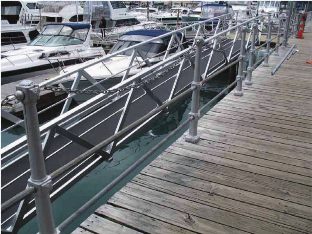
Modern balustrade incorporating recycled stations, Pier 21.
